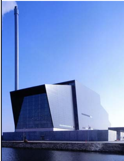
Danish waste-to-energy plant
