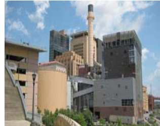
The District Energy Plant St. Paul. MN
