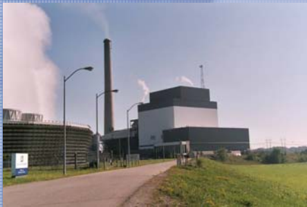
Ottumwa Generating Station, Iowa
